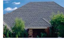
Stone Coated Steel Roofing Systems is pressure formed aluminum-zinc alloy coated steel with an acrylic bonded stone chip finish. The stone coating resists fading and UV penetration. For more information, contact one of our Goldin Metals locations.
